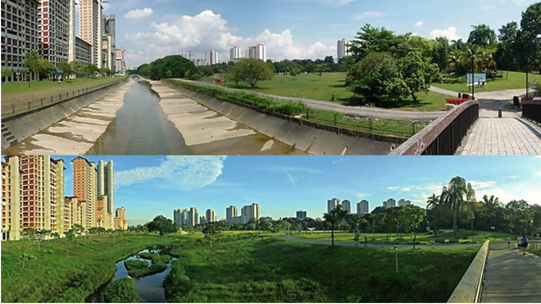
Water and Sustainable Design, Fig. 7 The critical shift from gray to blue-green infrastructures in Bishan-Ang Mo Kio Park, Singapore, in 2008 and 2013. (Photo Credit: Atelier Dreiseitl)
