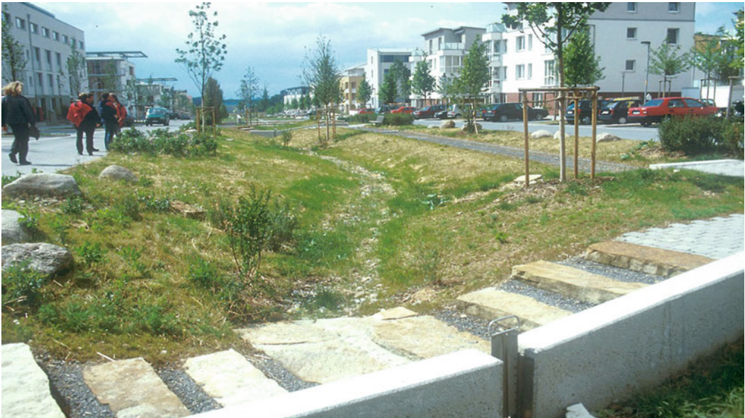
Water and Sustainable Design, Fig. 10 Hannover-Kronsberg, Germany, uses ecological BGI solutions to enhance urban and sustainable living. (Photo Credit: Herbert Dreiseitl)
