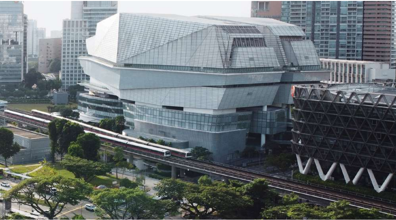
Buona Vista MRT Station in Singapur
