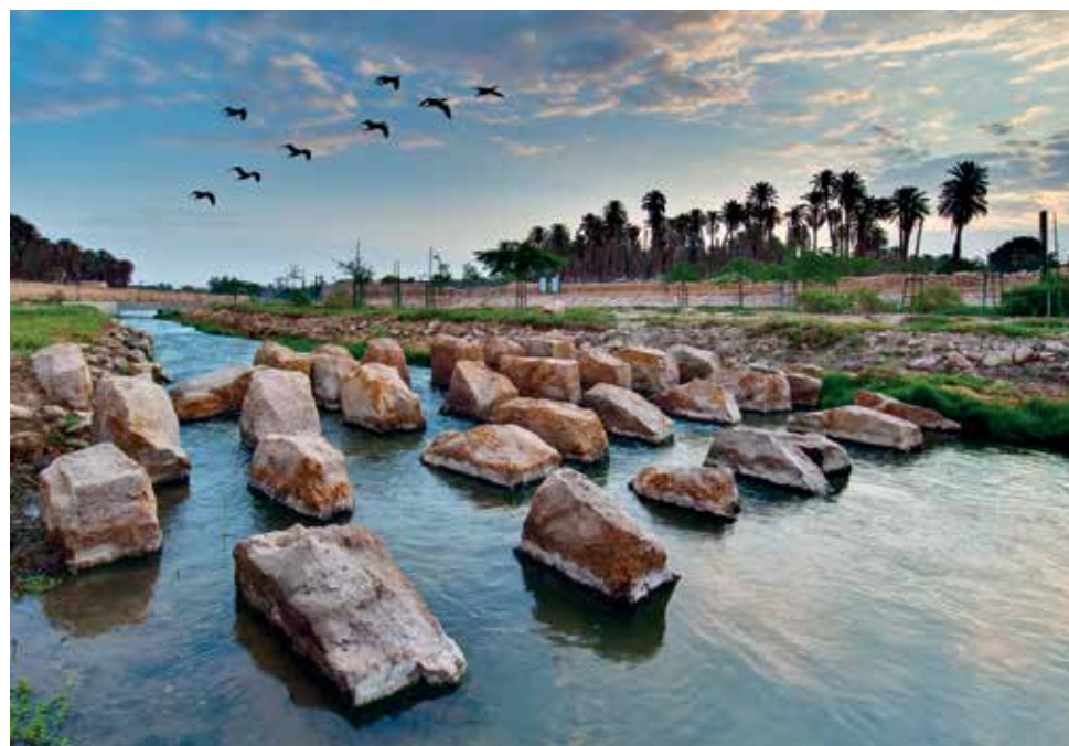
FIGURE 1: The Wadi Hanifah's naturalized channels employ check dams to attenuate water flow (bottom)
